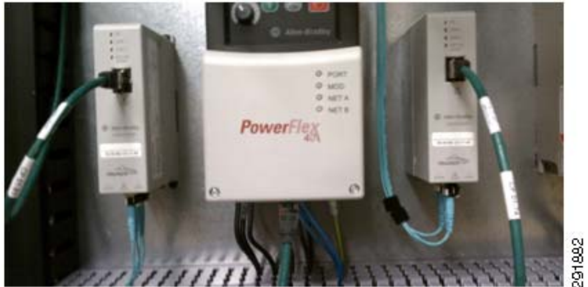
Figure 5 Sample Device-Level Fiber Optic Deployment
