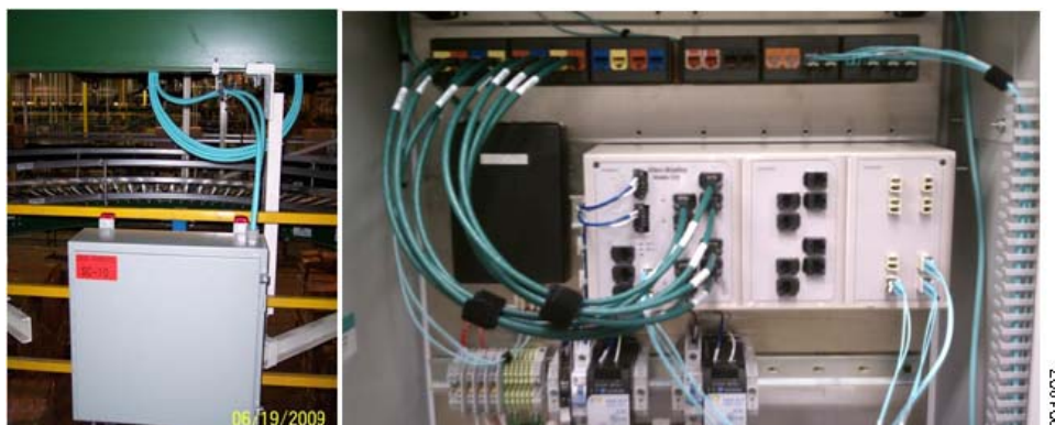
Figure 11 Sample Network Zone Fiber Optic Deployment
