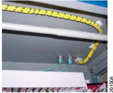
Figure 23 Armored Cable Bulkhead into Enclosure
